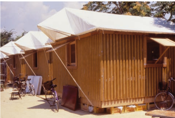
Abb. 2: Paper Log House, 1995, Kobe, Japan; Photo by Takanobu Sakuma
