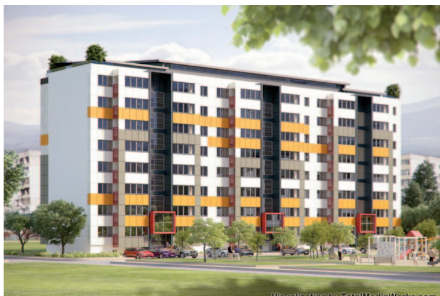
Fig. 5: New treatment of entrance areas and integration of social functions (a multifunctional space is designed above entrances)
