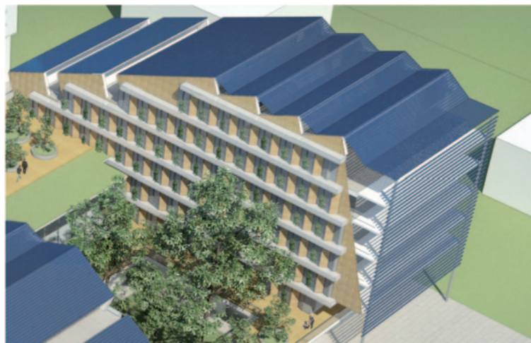
Fig 5: Integration of vacuum tube collectors in the south façade (Source: FUTUREbase Final Report, 2012)
